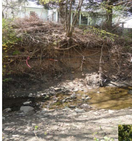
Top: Scotts Level Branch (Gwynns Falls Watershed) before stream restoration
