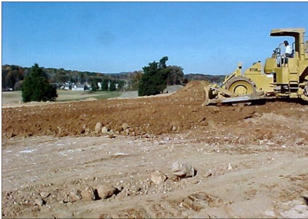
Figure 3: Excavation/Earth Moving Equipment (Photo courtesy of www.co.monterey.ca.us/.../grade/grading_powerpoint_060805.pps )
