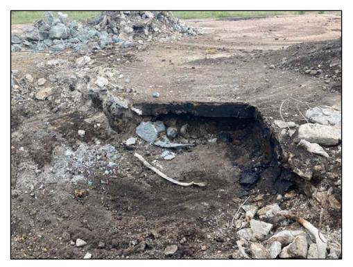
052920-5: Petroleum impacts observed in the northeastern corner of the B17-019-SB excavation area. Impacted material had a faint odor and was removed from the excavation.
