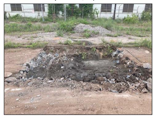
052920-2: B17-016-SB excavation area excavated to approximately 2 ft bgs, where a concrete structure was revealed.
