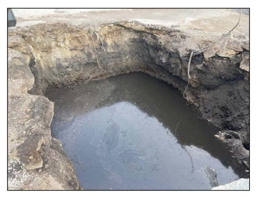
052920-1: B17-008-SB excavation area was excavated to approximately 8 ft bgs. Groundwater observed with a depth of 2-3 ft from the bottom of the excavated area.
