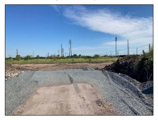
062620-1: Backfilling of B17-019-SB excavation area.
