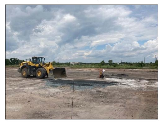
061920-3: Backfilling of B17-008-SB excavation area.
