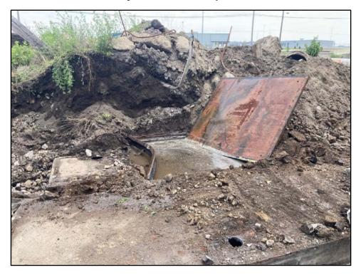
052920-4: A vault uncovered in the southeast corner of the B17-019-SB excavation area. Water in the vault was removed with a vacuum truck.
