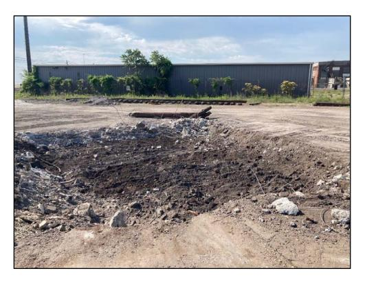
060220-3: B17-014A-SB excavation area was excavated to approximately 2 ft bgs. Rebar from the removed concrete foundations was observed around the excavation.
