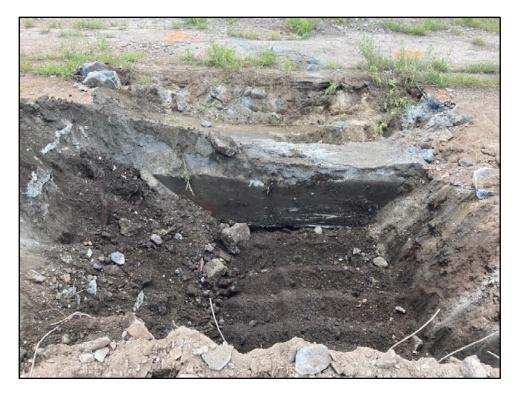
052920-3: B17-016-SB excavation area was excavated to approximately 4 ft bgs. Concrete pipe observed at 2 ft bgs.
