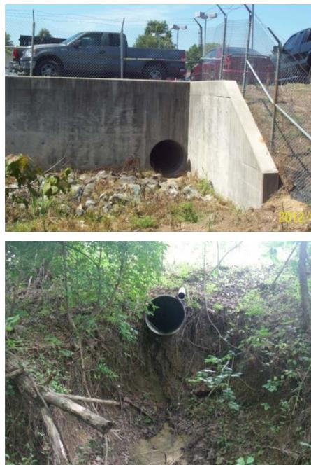
**Figure B.1.** The above outfalls are examples of locations that should be identified on storm drain maps and included in the permittee's screening program. Areas with highly developed land uses (e.g., commercial business complexes, aging infrastructure) have a greater potential to pollute and should be prioritized. Structural stability and erosion concerns should also be identified and corrected as part of an effective IDDE program.
