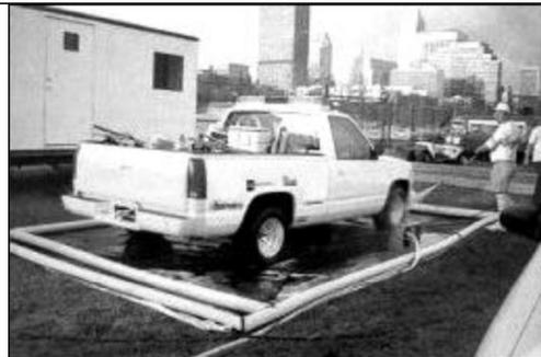
Figure 6 - Containment System Preventing Wash Water from Entering the Storm Drain
