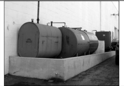
Figure 15 - Secondary Containment of Storage Drums behind a Car Repair Shop
