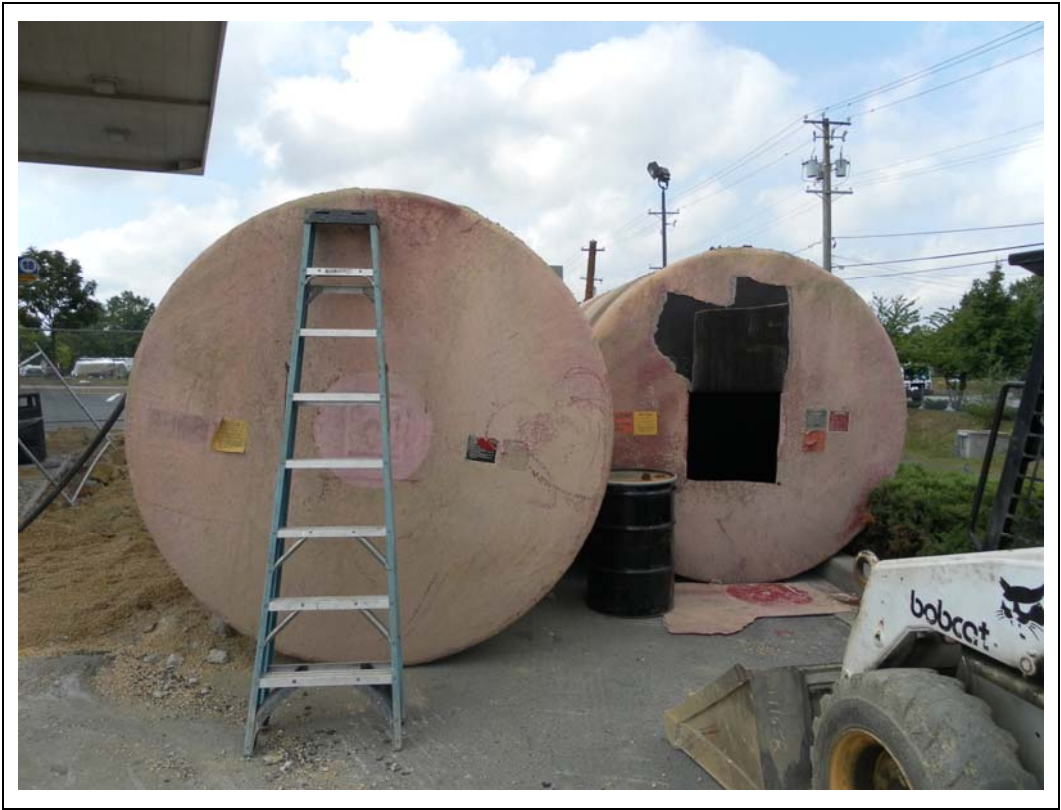
Photograph 1: View of former 12,000 gallon diesel UST open for cleaning.
