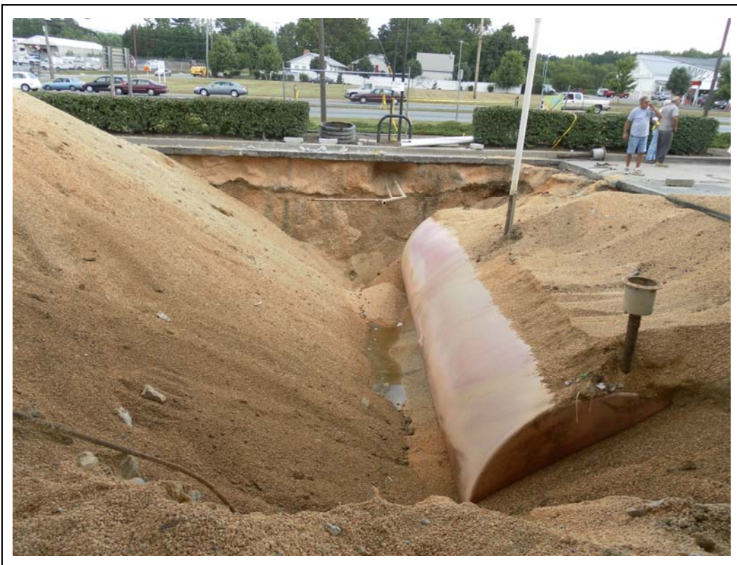
Photograph 4: View of the partially uncovered 20,000-gallon regular unleaded UST from the south.
