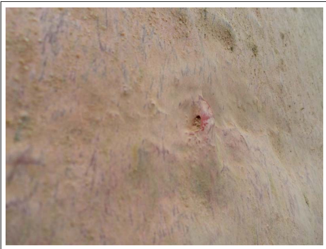
Photograph 8: View of suspected pinhole in FRP secondary containment (south end of tank).
