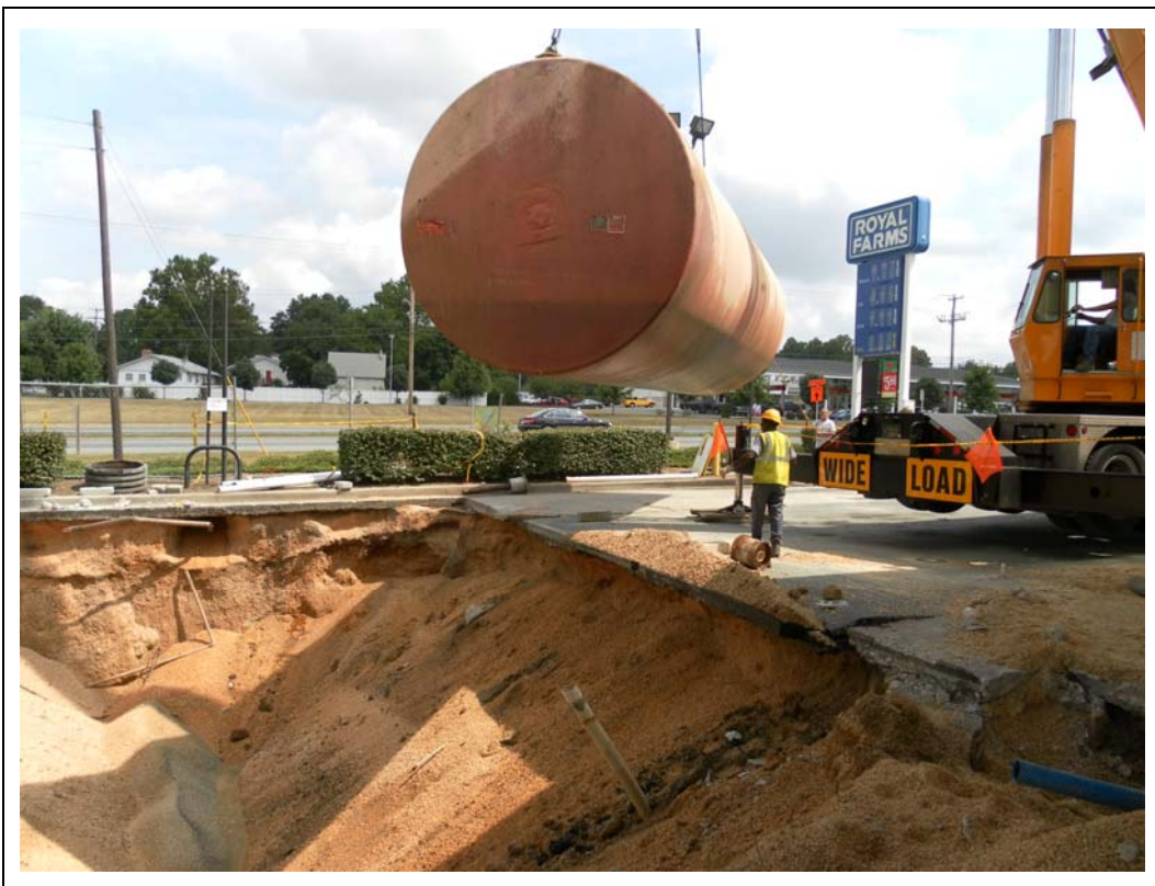
Photograph 6: Additional view of the 20,000-gallon tank being removed by a crane.
