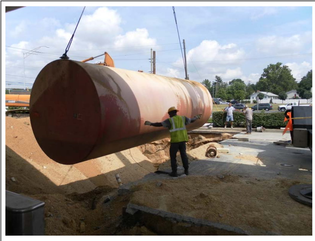
Photograph 5: View of the 20,000-gallon UST being removed from the tank pit excavation.
