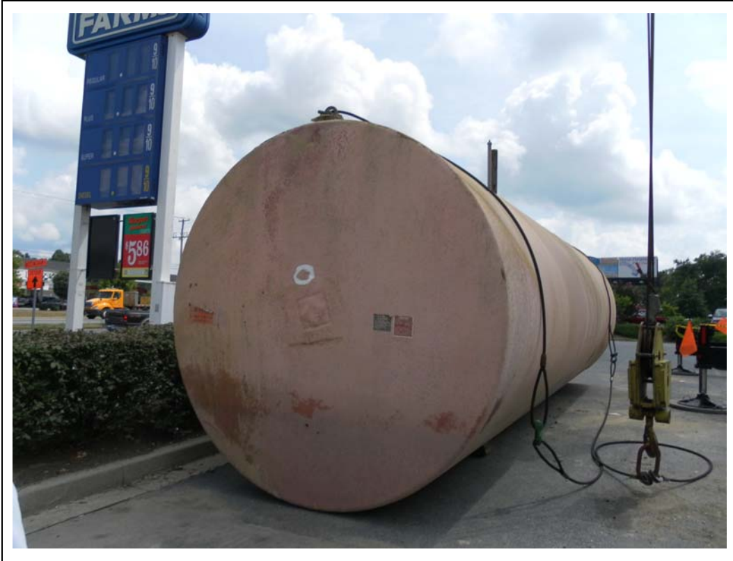
Photograph 9: View of the southern side of the 20,000-gallon UST (suspect pinhole circled in white paint).
