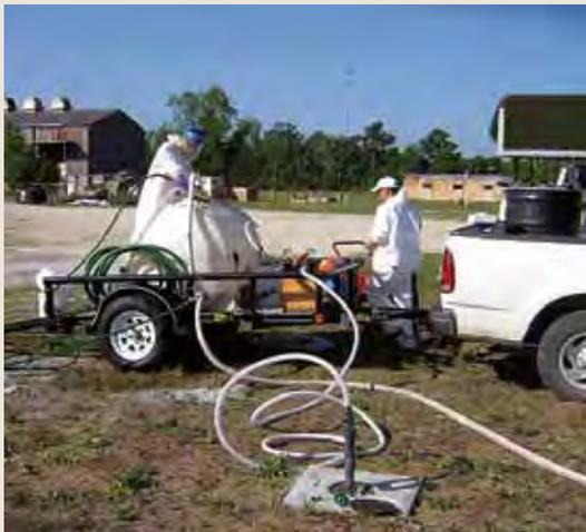
FIGURE 2: 3-D MICROEMULSION IS TYPICALLY APPLIED THROUGH PERMANENT WELLS OR BY USING DIRECT-PUSH INJECTION
