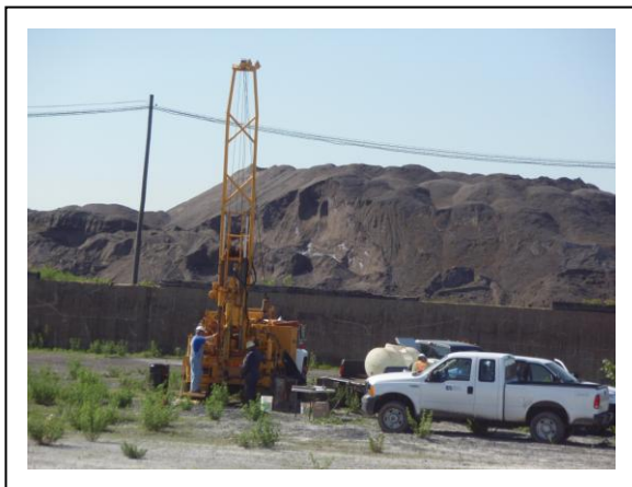
Figure 1. Drill rig setup with hollow stem auger
