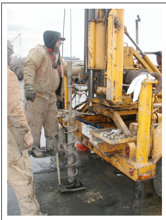
Figure 3. Drilling sediment cores
