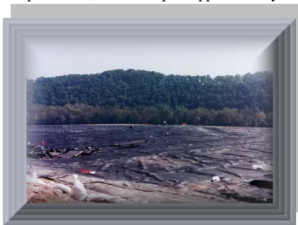
Landfill Liner Installation.
